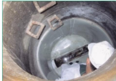
Sewer manhole lined with Carbofix® and the modular connection.
