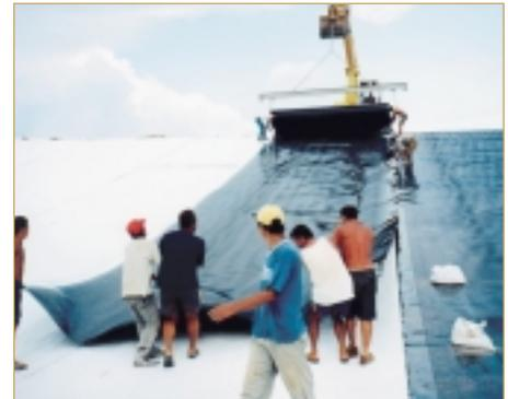
Installing a composite lining system using Carbofol® on top of Bentofix®
