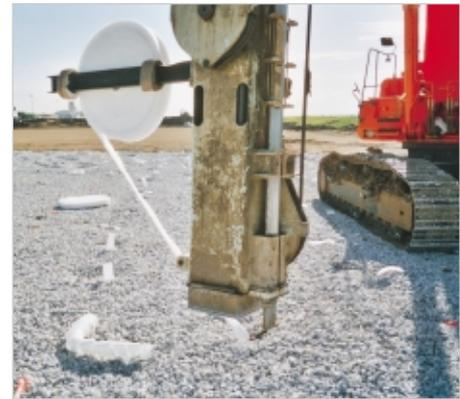
Excavator inserting Secudrän® V through the load-bearing layer
