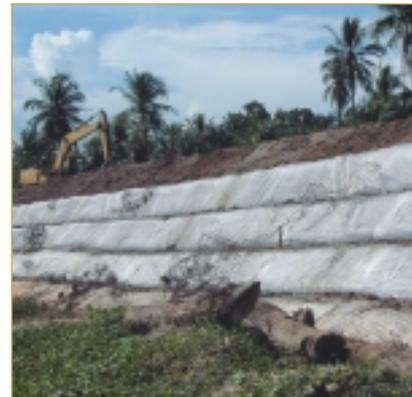
Secugrid® as embankment reinforcement
