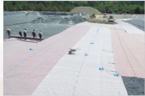
Installing Secutex® on the Carbofol® geomembrane, and the placement of a mineral drainage layer
