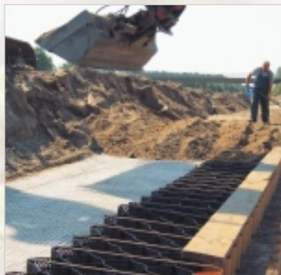
Filling of the Secugrid® reinforced geocells
