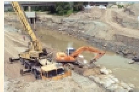
Installation of Secutex® Sand containers as down stream dam to capture sediments
