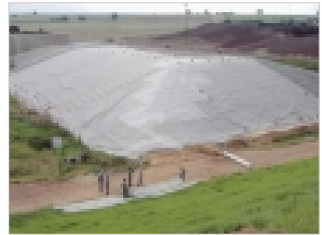
Installation of 1.5 mm Carbofol® geomembrane
