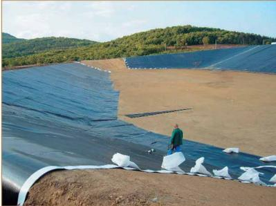
Carbofol® KDB installed as base sealing system
