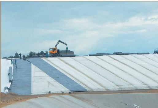
The basis sealing comprising Carbofol® KDB installed over GTD Bentofix®
