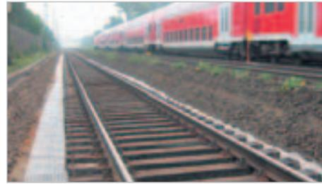
Secugrid® geogrid laid beneath wooden ties and SPL
