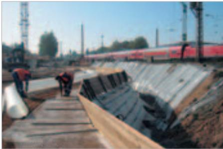
Secugrid® geogrid installation in the embankment slope
