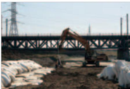
Placing of soil filled Secutex® scour protection sandcontainers
