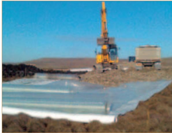
Placement of crushed gravel base course over the installed Secugrid® reinforcement
