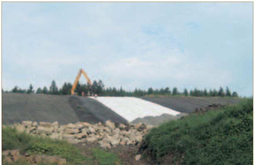
50 cm thick mineral clay liner as listed in the tender. The selected needle-punched GCL has a high swelling bentonite powder sealing layer, high interface and internal shear properties and is considered as an approved alternative to CCLs. It has also been rated positively by German LAGA Ad-hoc-AG "Deponietechnische
