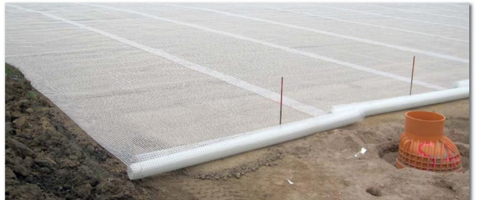
it possible to site the biogas plant there. Installed within a 450mm thick crushed rock subbase (200mm and 250mm) underneath a 650mm thick superstructure, the geogrid reinforcement contributed significantly to the fact that the foundation became a real load-bearing layer.
