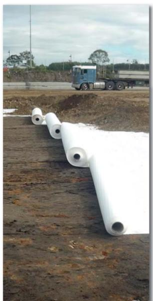
environmental advantages of construction methods with geosynthetics, especially on soft soils are already well known. Soil masses that need to be excavated, transported and installed can be dramatically reduced by the inclusion of geosynthetics. The best example is the improvement of soft subgrades with geogrids or geocomposite products. Geotextiles are normally required to separate a granular platform from a cohesive subgrade and to act as a filter.
